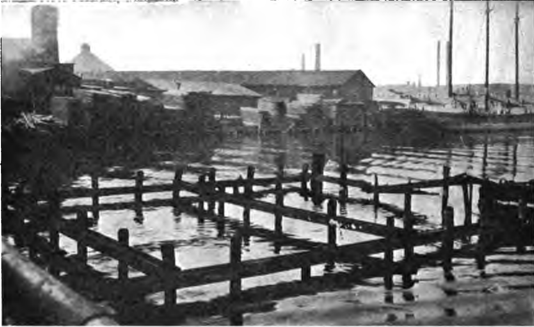
West Shore Pequonock River looking north from Washington Avenue Bridge, Bridgeport
